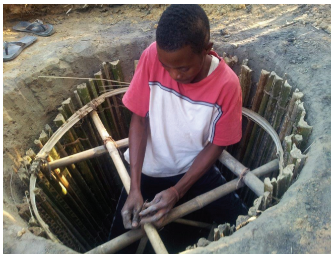
A community worker lines and reinforces a latrine wall with local materials in Katanga, DRC. Photographer: Chaungo Barasa (2013)
